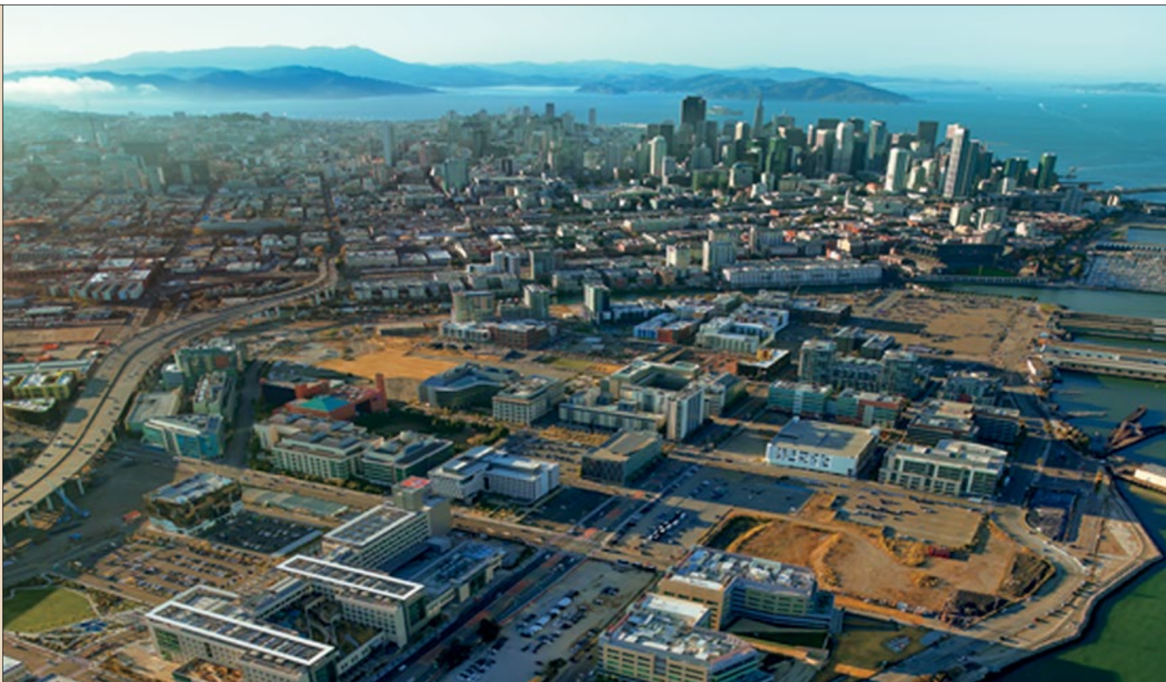
New home for Ophthalmology at Mission Bay – in the heart of UCSF's biotech campus.
